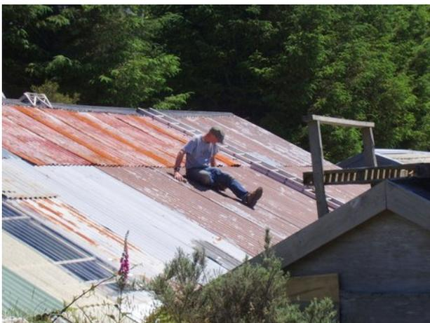
Also on site was Shige Ohashi measuring and making templates for formers to be used in supporting the roof of the kiln while repairs are undertaken. Over the course of 10 firings the roof has slumped a little. Firewood processing has also started.
